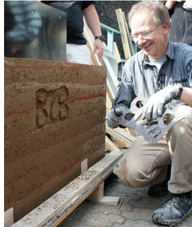
Fig. 3 Rammed earth element, DVL Specialist for Earth Building (FKL)
