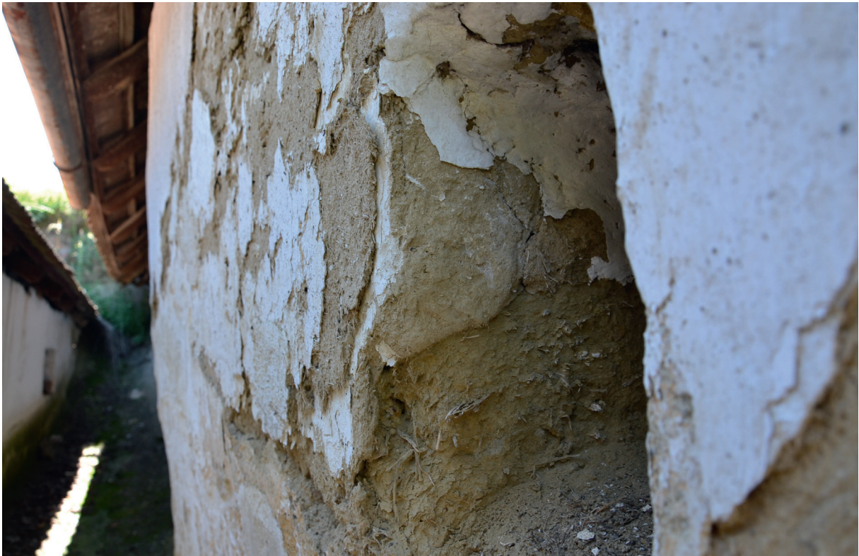
Fig. 4 "G'satz" masonry in Haugsdorf (Lower Austria)
