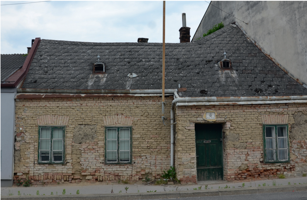
Fig. 8 Historical mixed masonry in the urban environment of Hollabrunn (Lower Austria)
