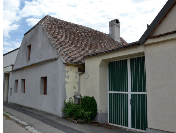
Fig. 10 Restoration with inappropriate materials: EPS exterior insulation of a historical earth block building in Lower Austria
