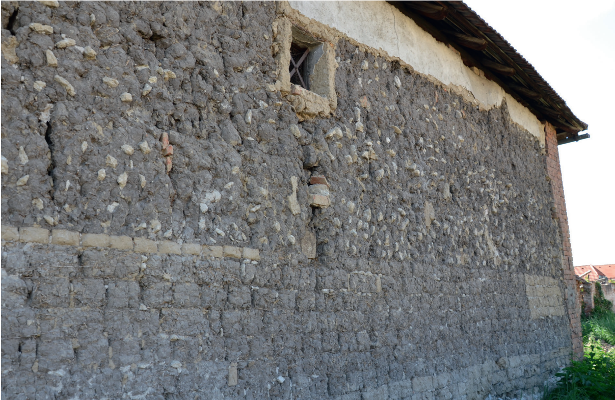
Fig. 5 “Wuzel” masonry built on ashlar masonry in Zellerndorf in Lower Austria
