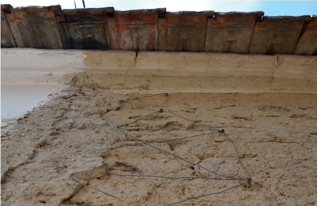
Fig. 3 Exterior plaster layers of a Weinviertel earth block house with whitewash
