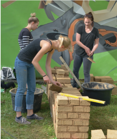
Fig. 1 Building with adobe bricks on the 1st Eco-Building Day at Wismar University of Applied Sciences in 2014
