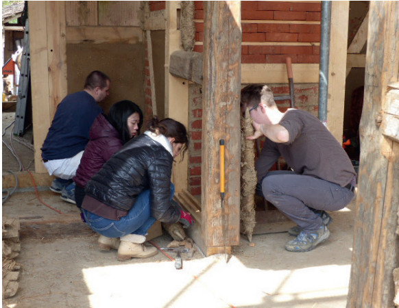
Fig. 4 Working on the building site: fitting wattles into the timber structure
