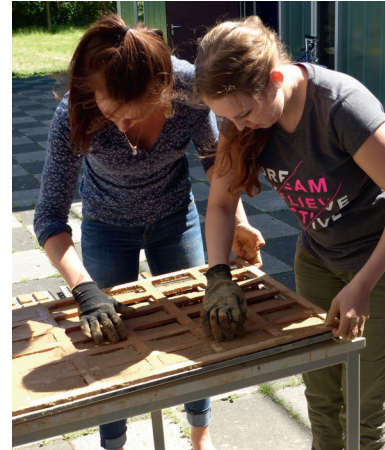
Fig. 3 Making clay tiles for the construction of a Catalan vault on the Campus of Wismar University of Applied Sciences as part of the 3rd Eco-Building Day in 2016
