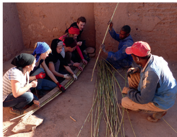
Figs. 8 + 9 Working together with and learning from locals: Making a ladder of bamboo on Lake Agege Farm in Ghana; Weaving a reed mat for the renewal of a ceiling in the Tamnougalt Casbah in Morocco
