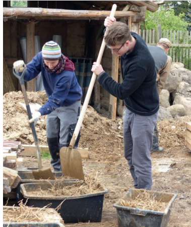
Fig. 2 Working on the building site: mixing mortar
