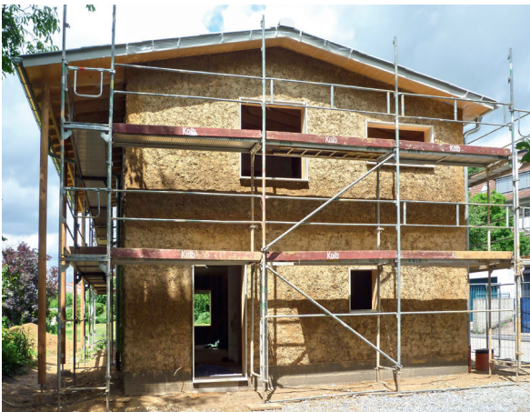
Figs. 3-6 Haus J, Darmstadt. 3: Completed building after a construction period of six months: the shell of heavy straw light earth is coated with a lime render. 4: The continuous earth shell enveloping the house took approximately four weeks to dry out. 5: Timber structure with a lattice of battens onto which the light earth is applied. The roof protected earth construction works from the weather. 6: Preparation of clay slurry from dry earth with a Knauf PFT G4 mixing machine.
