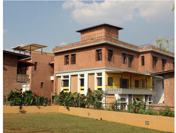
Fig. 7 Exposed CSSB masonry buildings
