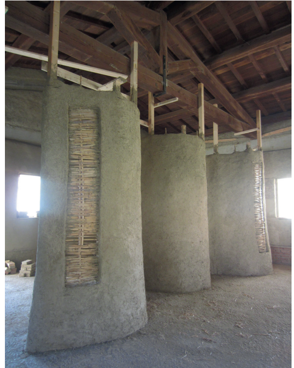
Fig. 7 Interior partition as a wattle and daub structure
