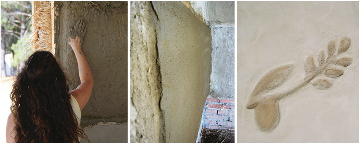
Fig. 9 The three layers of the plaster
