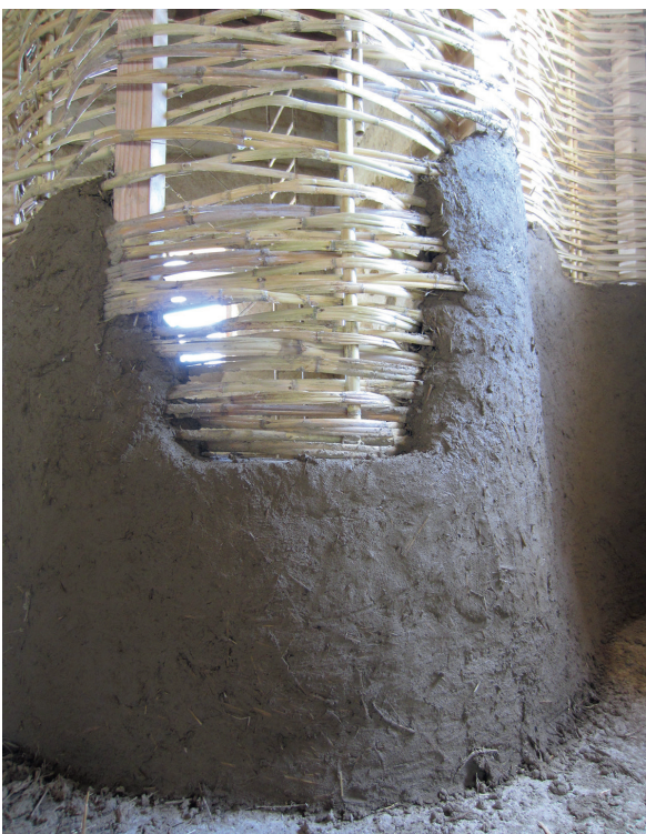
Fig. 10 Detail of the wattle and daub wall
