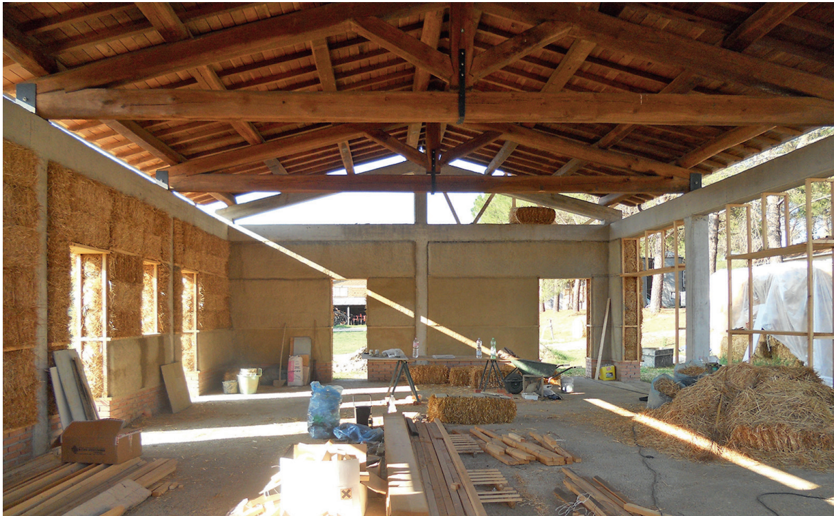
Fig. 5 The different stages of the construction: concrete structure, timber substructure, straw bale wall and clay plaster
