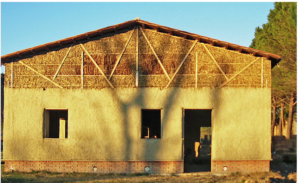
Fig. 8 In construction: the straw bale walls, clay plaster and light earth in the framework of the concrete structure
