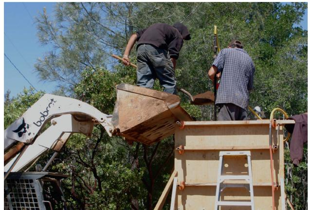
of man-hours to accomplish the task. A slightly faster method utilizes shovels for proportioning and a small garden roto-tiller for blending. Faster still is a small front-loading tractor, which can both proportion and blend, with water added as needed with a garden hose. Tractor mixing can be made more efficient and more thorough with a tiller mounted on the back.
