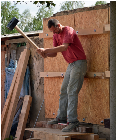
Fig. 7 Hammering in the steel plates beneath the wall
