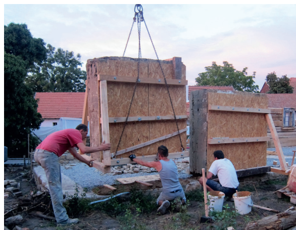
Fig. 10 In Přerov nad Labem: the wall sections are seated on a new, pre-built wall base, September 2015
