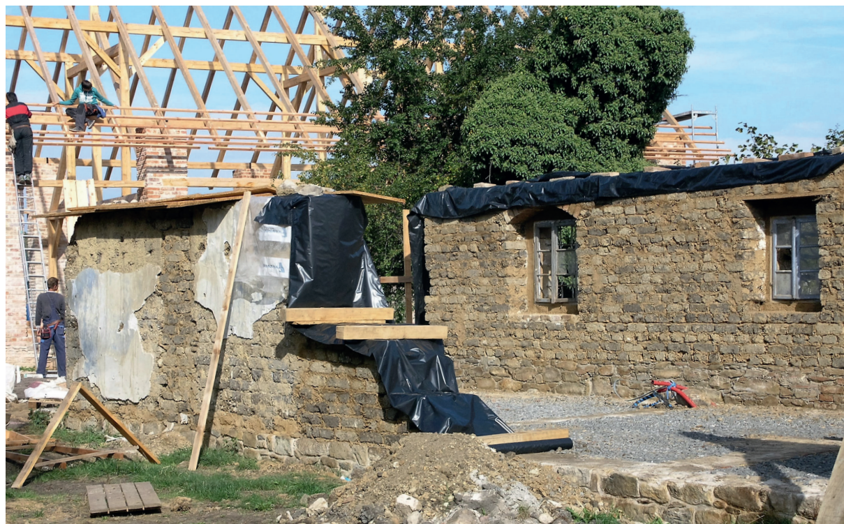
Fig. 11 In Přerov nad Labem: the two walls sections are in the foreground, the stabilised block with the cracks on the right. In the background, the newly built courtyard wall made of transferred original unfired bricks. September 2015.
