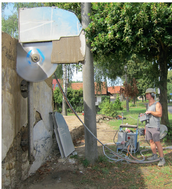
Fig. 5 Cutting of the earth wall to the store room on the street facade with a water-cooled diamond circular saw
