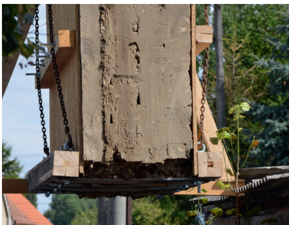
Fig. 9 Detail of the construction of the formwork, the bearing steel plates and the supporting brackets
