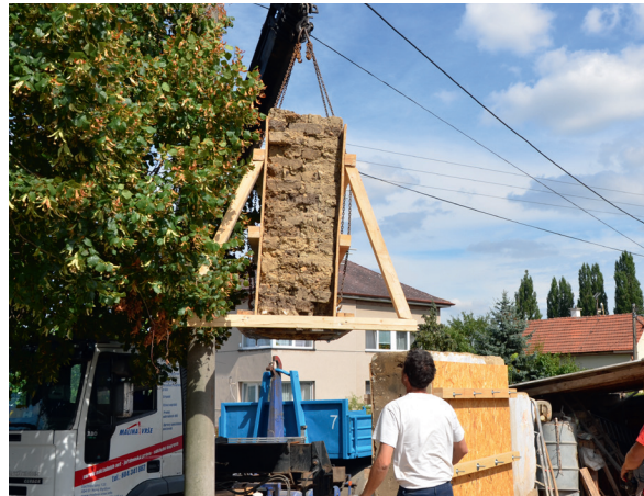
Fig. 8 Transfer of the first block with a hydraulic crane arm. Cracks are visible in the wall.
