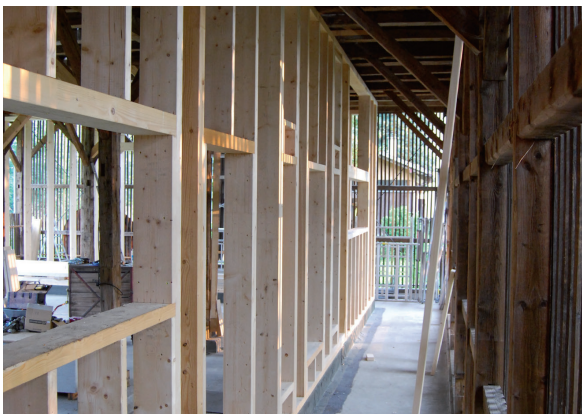
Fig. 12 Reversible timber constructions in both the new and old parts of the “Torfremise” in Schechen
