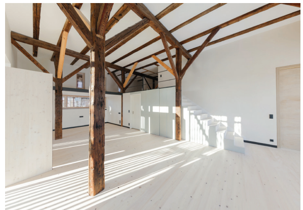
Fig. 12 Reversible timber constructions in both the new and old parts of the “Torfremise” in Schechen
