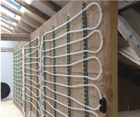
Fig. 11 Wood and earth wall with wall-heating pipes prior to embedding in clay plaster (Torfremise)
