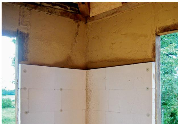
Since the exposure to dampness of an external wall from the outside due to weathering is 150 times greater than from inside through diffusion, the condition of the exposed external wall should also be checked. Cracks or open joints at junctions can present the risk of excess moisture ingress from outside. With timber frame constructions, one should also examine high gables or wall areas because wind loads can also lead to increased moisture ingress.
