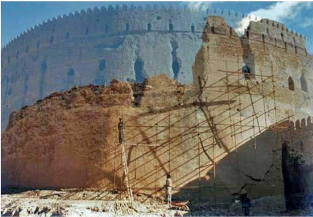
which prevents the mud blocks from fracturing. In addition, in Iranian vernacular architecture, wood powder was also added to the mud in order to increase its tensile strength and resistance. Gradual deterioration of the wood and eradication of straw by termites have resulted in the removal of the stabilising materials in adobe structures (wood) as well as elimination of the strengthening agent against tensile forces (straw).
