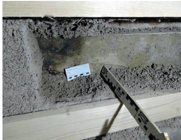
Fig. 4 a + b Mould and fungus formation due to too slow drying of the light earth internal insulation layer. Mill, Germany
