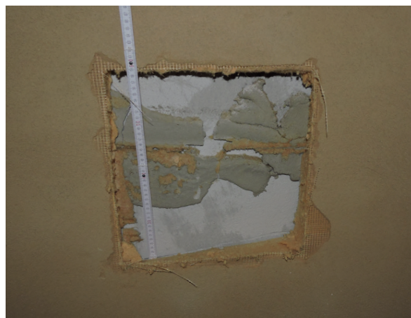
Fig. 5 a + b The improper bonding of the internal insulation panels could be detected by knocking and is plainly visible at open junctions such as the window sill. After opening a section of the wall, the full extent of the inappropriate bonding method was revealed.
