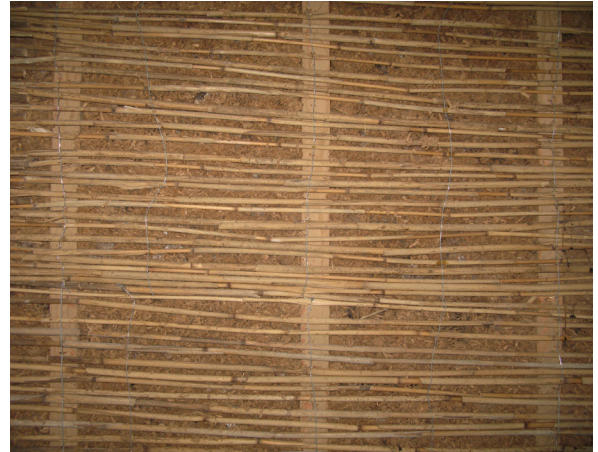
Fig. 6 a + b Light earth internal insulation with hemp. Former livestock barn in Ribbeck, Germany
