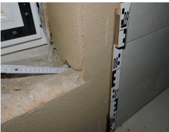
Fig. 5 a + b The improper bonding of the internal insulation panels could be detected by knocking and is plainly visible at open junctions such as the window sill. After opening a section of the wall, the full extent of the inappropriate bonding method was revealed.
