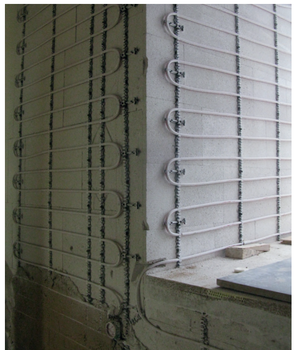
Fig. 7 a + b Internal insulation of a granary in Freiberg/Saxony (Germany) with mineral foam insulation board bedded in earth mortar with additional wall heating and clay facing plaster
