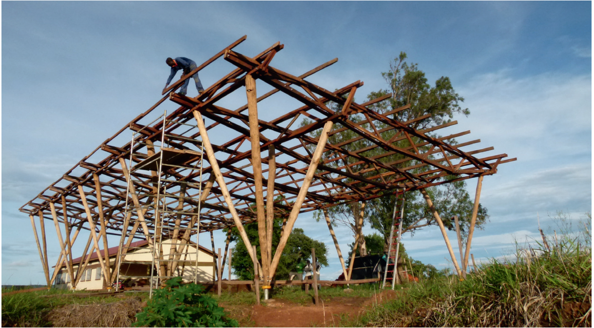
Assembling the roof structure
