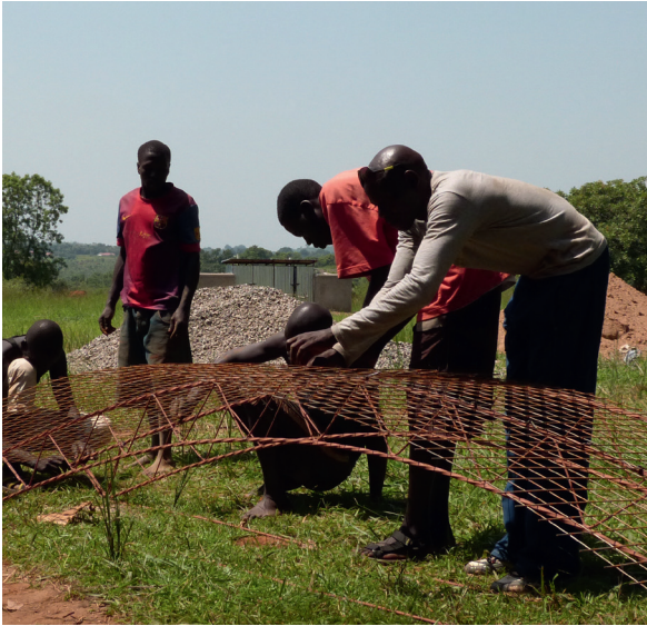
Pre-fabrication of the ceiling elements
