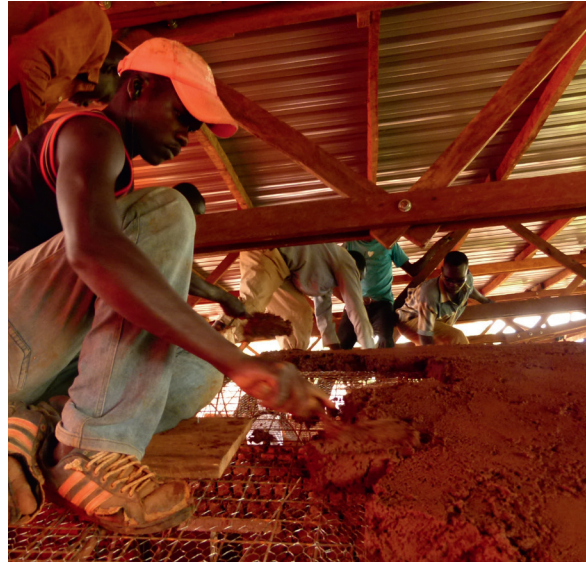
Application of daub onto the ceiling elements
