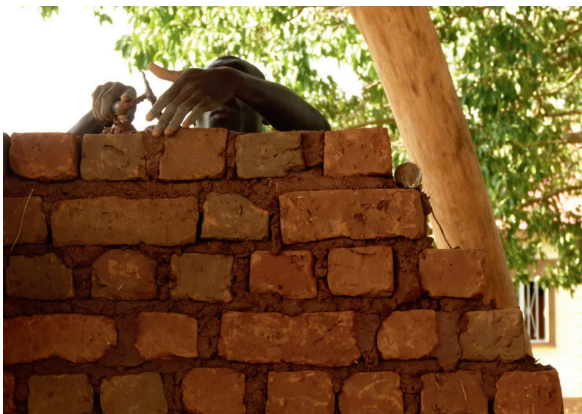
Mason Ogwal laying earth blocks
