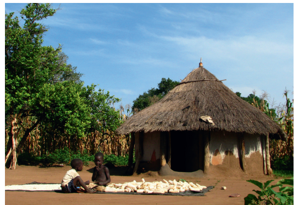
Traditional tukul with externally-placed wooden posts
