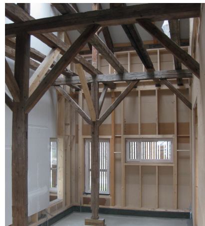
Fig. 10 External walls of the new insertion as a highly-insulated skin
