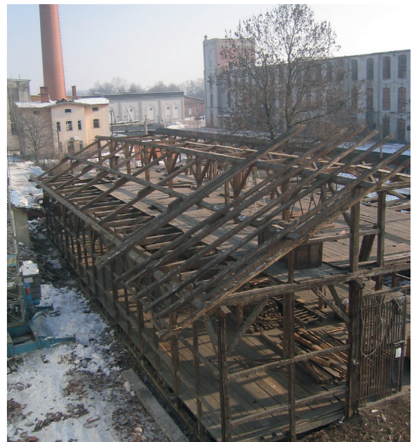
Fig. 2 Dismantling and removal of the building from the spinning mill site in Kolbermoor
