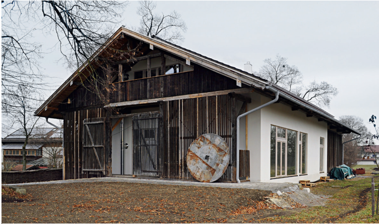
Fig. 5 House-in-house: the volume of the new insertion protrudes beyond the frame of the old building
