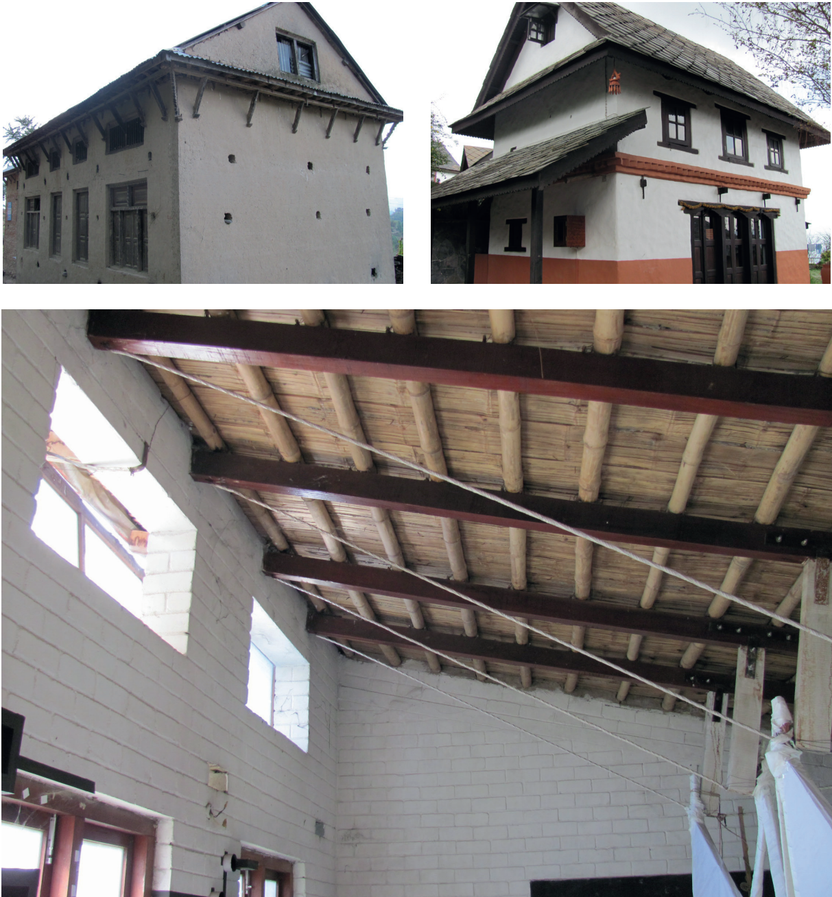
Fig. 11 - 13 Modern adaptation of the Newar Style which can be seen throughout the valleys of the Kathmandu. Model house at Tribhuvan University in Kathmandu made of compressed earth blocks (made with an AURAM earth block press) with an innovative construction method for reinforcing the structure against seismic forces. Project led by Prof. Dr. Sushil B Bajracharya, Associate Professor at the Department of Architecture and Planning, Institute of Engineering (IOE), Tribhuvan University (TU)
